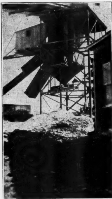
Chute and Housing For Grizzlies
